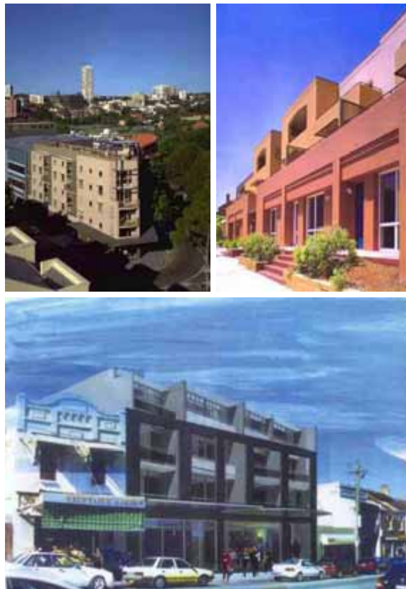
Figure 8: Indicative examples of the three building typologies: 100% BTL (top left), 80% BTL (bottom), 50% BTL (top right)
